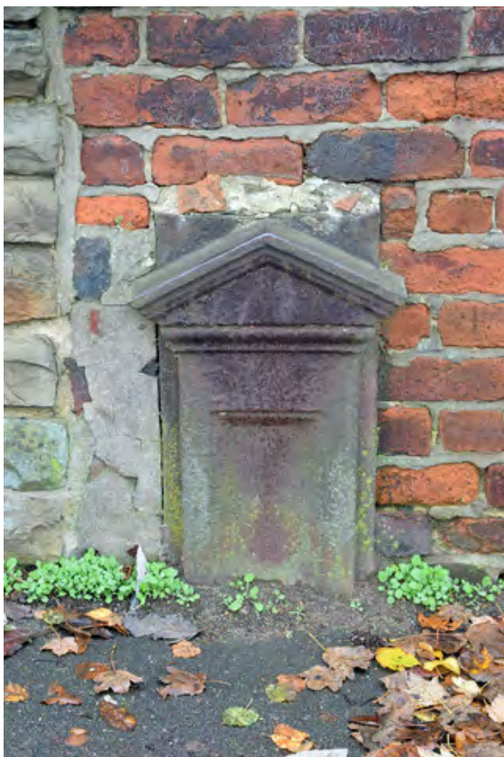
Former Brightside and Carbrook Co-operative store pilaster base No. 1 © Mike Higginbottom
