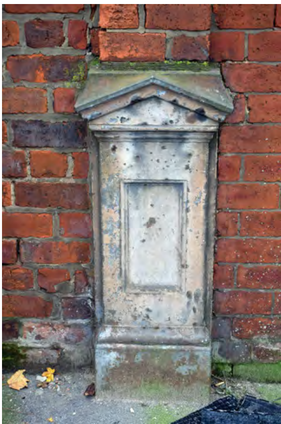
Former Brightside and Carbrook Co-operative store pilaster base No. 3 © Mike Higginbottom
