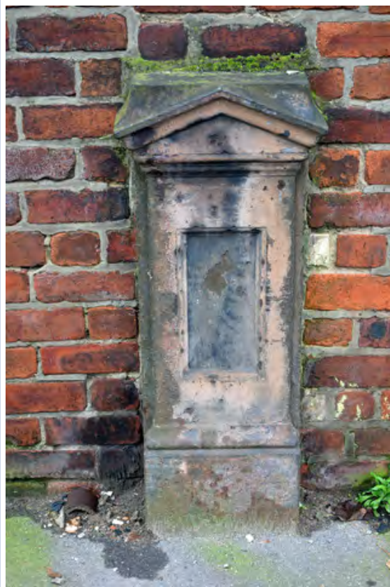
Former Brightside and Carbrook Co-operative store pilaster base No. 2 © Mike Higginbottom
