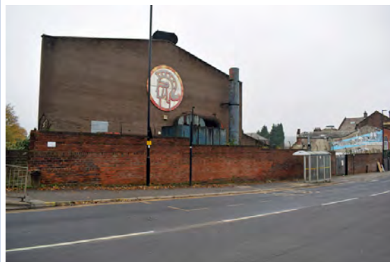
Former Brightside and Carbrook Co-operative store pilaster bases © Mike Higginbottom
