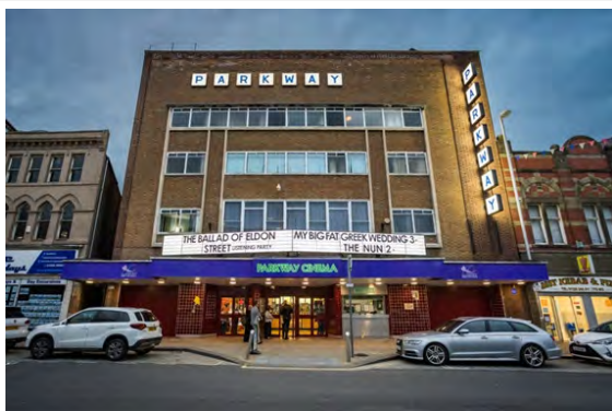
Parkway cinema frontage September 2023, showing reinstated signs and read-o-graph
