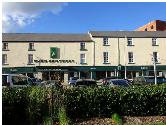
Harwood Terrace, showing a restored element.
