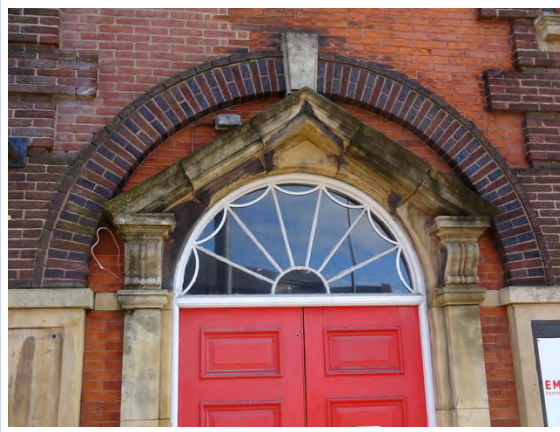
Detail of the fanlight above the York House entrance
