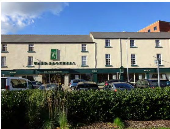
Harwood Terrace, showing a restored element.
