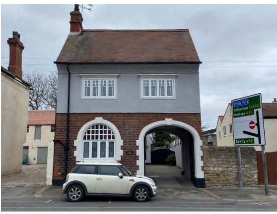
West facing elevation fronting onto Tickhill conservation area
