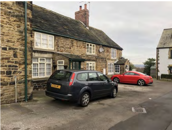
View of 5-7 Street, looking north-west
