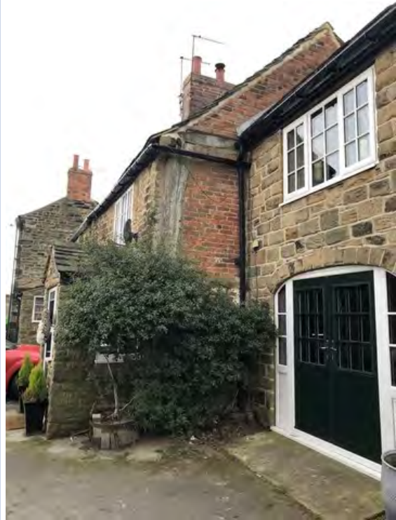
View of the north gable of 7 Street, showing timber framing.
