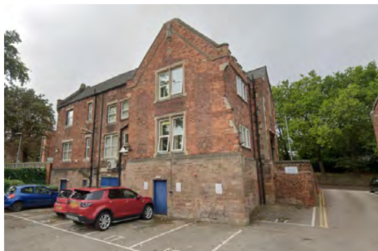
Rear elevation of the Former Grammar School
