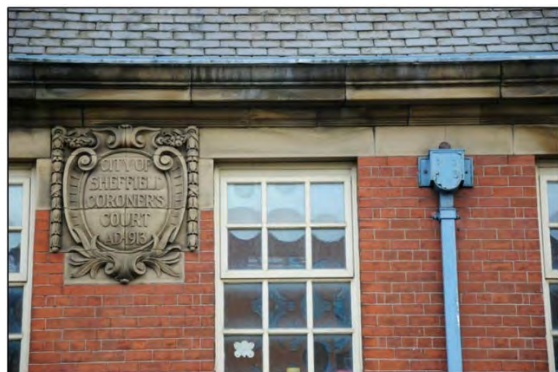
Date plaque on facade of the Old Coroner's Court
