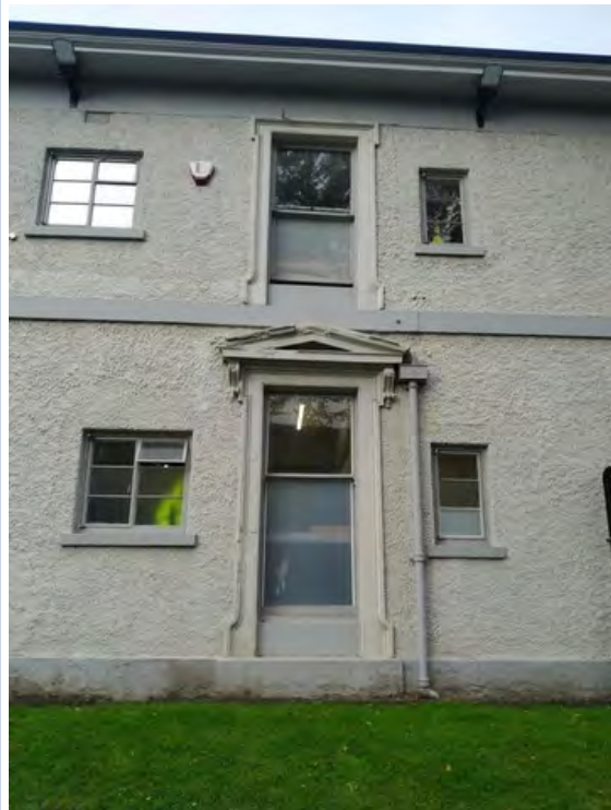
205 Brook Hill, detail from east elevation.
