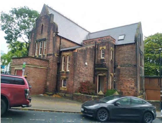
Westbourne Villa west elevation
