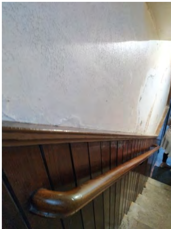
Worrall Chapel internal staircase
