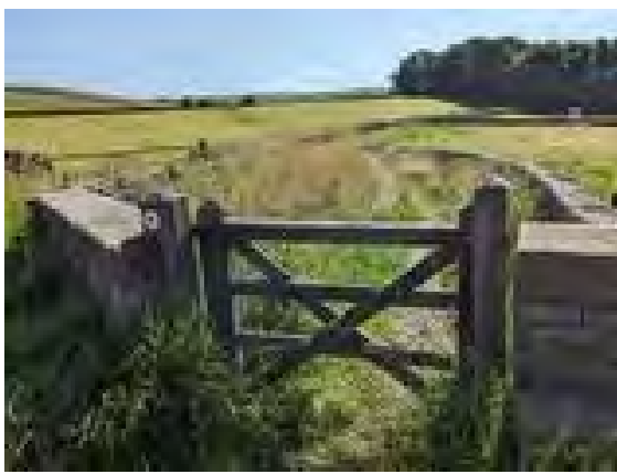
A view of the conduit running through fields close to its source.
